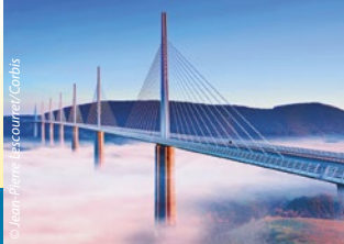
One of the highest bridges in the world - The Millau Viaduct (France).
